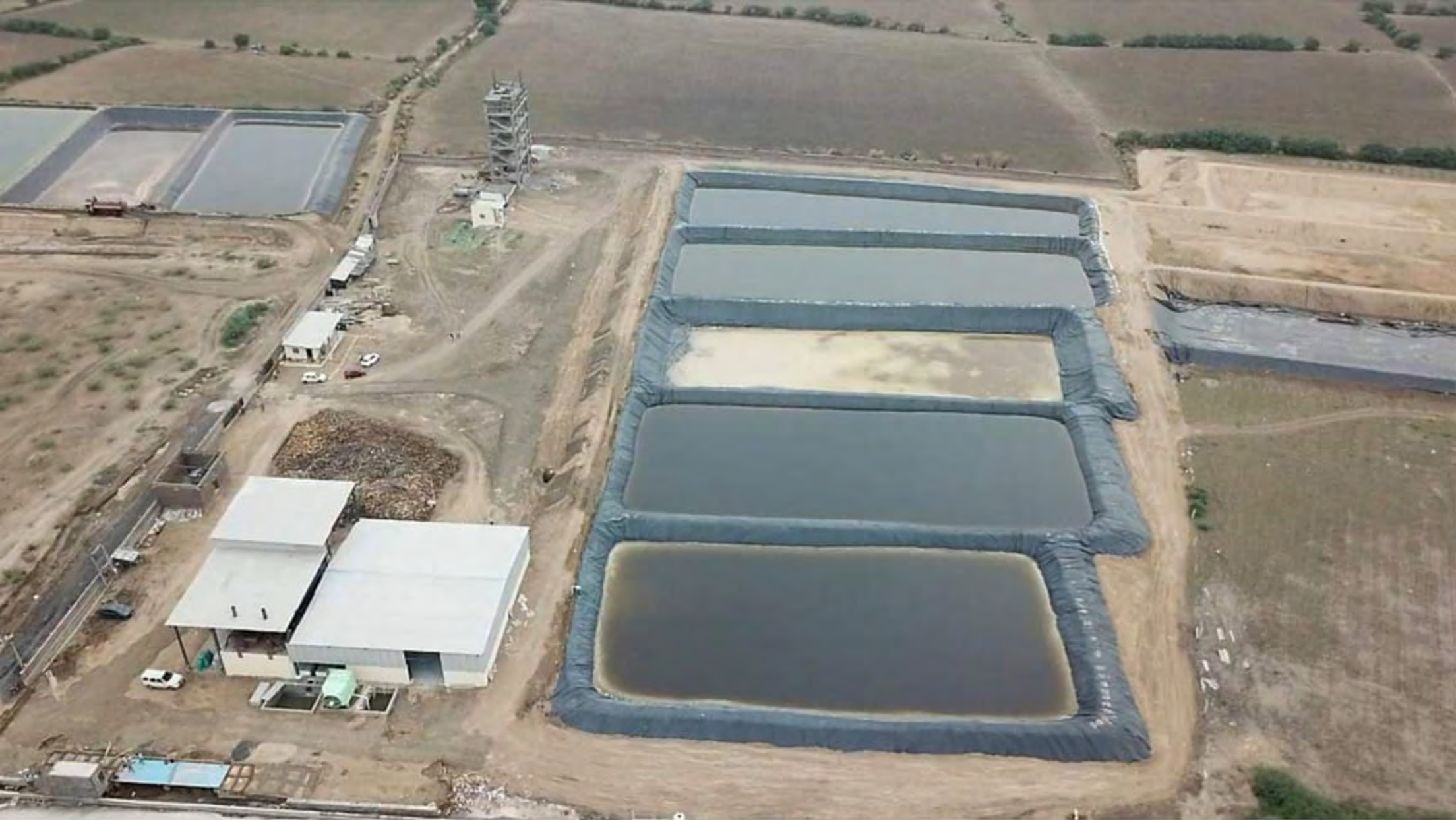
JHPL FACTORY SITE OVERVIEW
